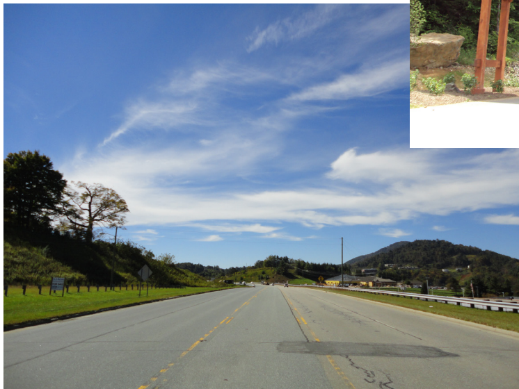
Left: Narrowing travel lanes, or adding additional corridor width during the next resurfacing project on US-421 would provide room for bicycle lanes.
