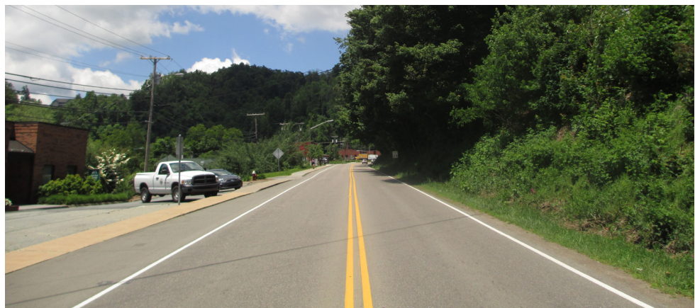
US-421 looking west out of town, with limited shoulder shown on the westbound side of the corridor.
