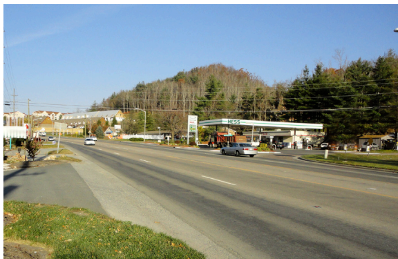
Left: Existing roadway conditions on NC 105, with two lanes in each direction and a center turn lane.
