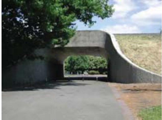
This undercrossing provides ample vertical and horizontal clearance and a clear sight line through the structure, improving the feeling of safety.
