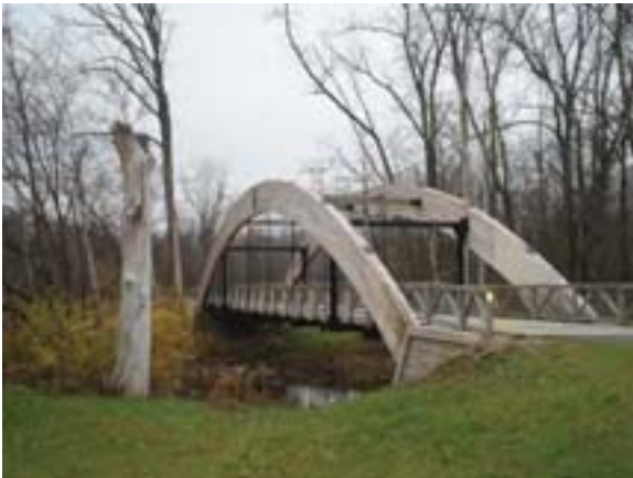
Bridge over Alum Creek
