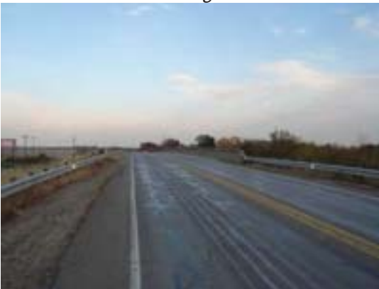
Bridge over railroad tracks
