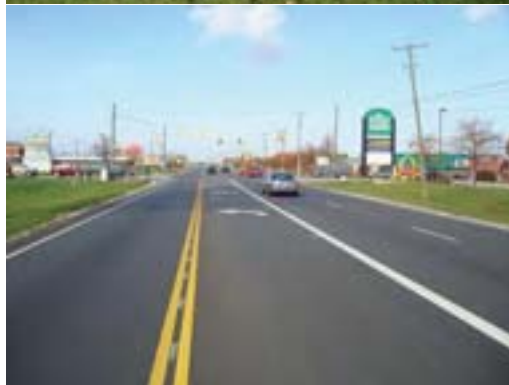
Typical cross-section of SR-161 in residential (far left) and commercial (left) areas.
