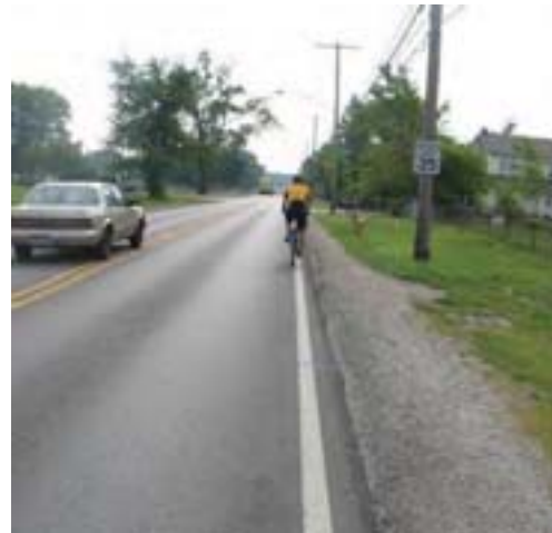
Paving the shoulder on this road would allow the bicyclist and motor vehicle to share the roadway
