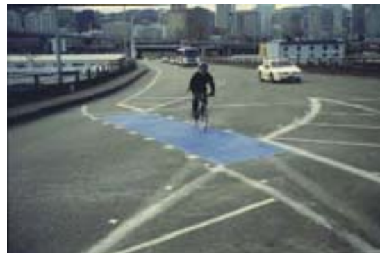
This blue bike lane in Portland is used to warn motorists approaching the on-ramp that bicyclists have a through lane.
