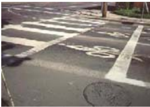
Bike box in Eugene, OR. (Photo: Evaluation of an Innovative Application of the Bike Box, FHWA, 2000.)
