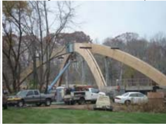
Construction of Broadmeadows Bridge to Olentangy Trail
