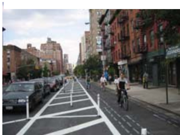
Example of a one-way cycle track from San Francisco Bicycle Plan Design Guidelines. 9th Avenue Cycle Track in New York City. Photo: www.streetsblog.org Oct. 5, 2007 post.
