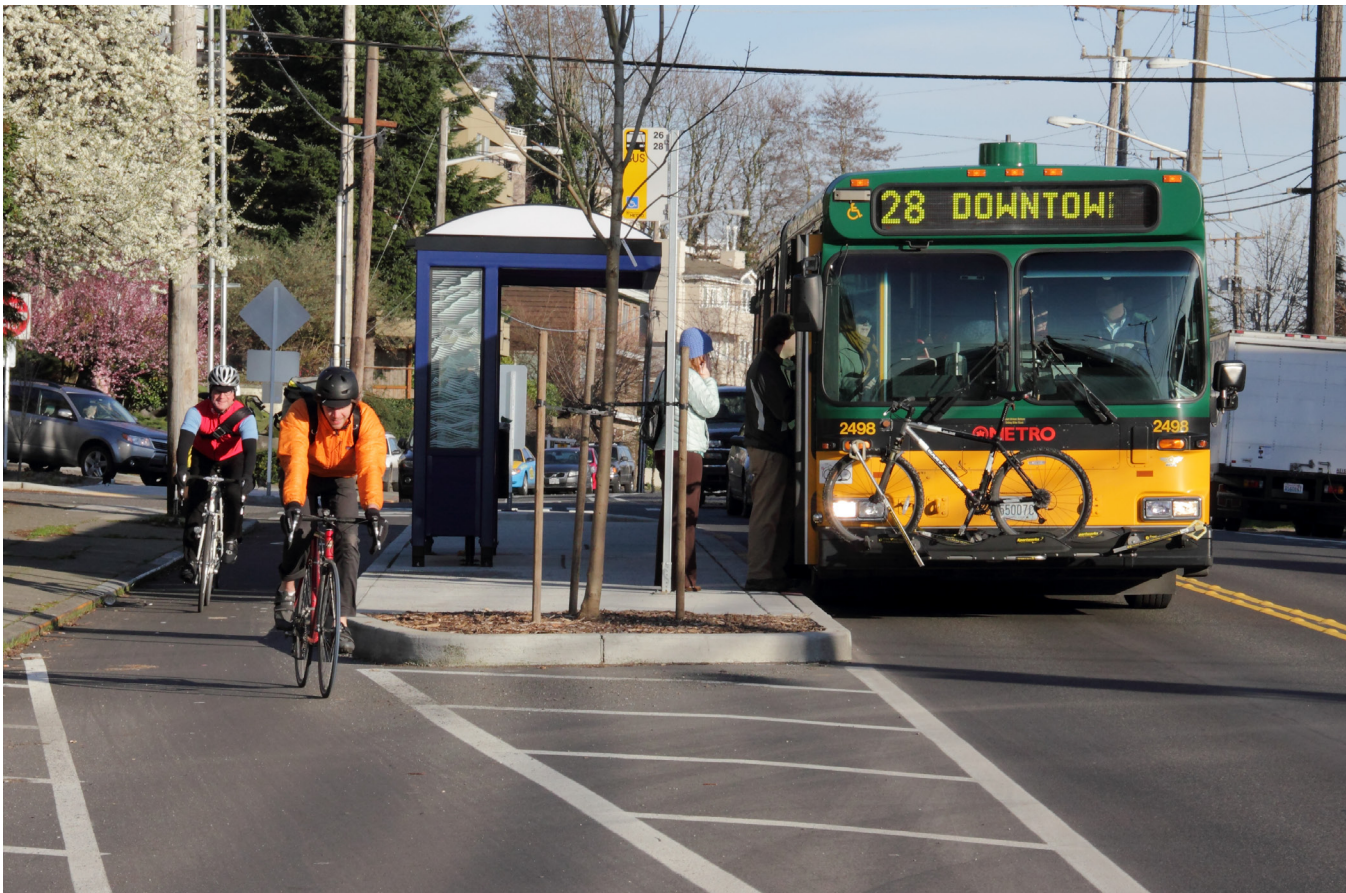
Buffered bicycle lane and transit island cycle track (protected bicycle lanes) on Dexter Avenue.
