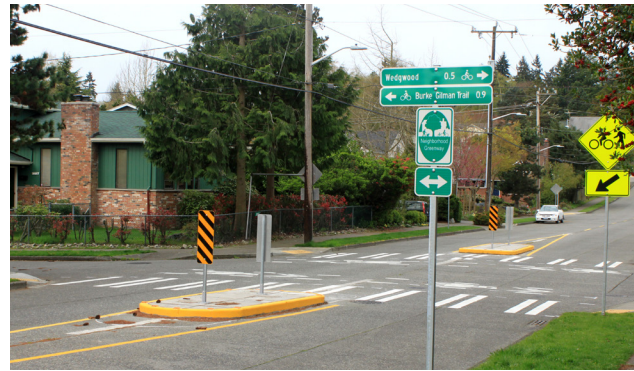
Wayfinding signs can promote bicycle facilities to potential riders and help people on bicycles get to their destination
