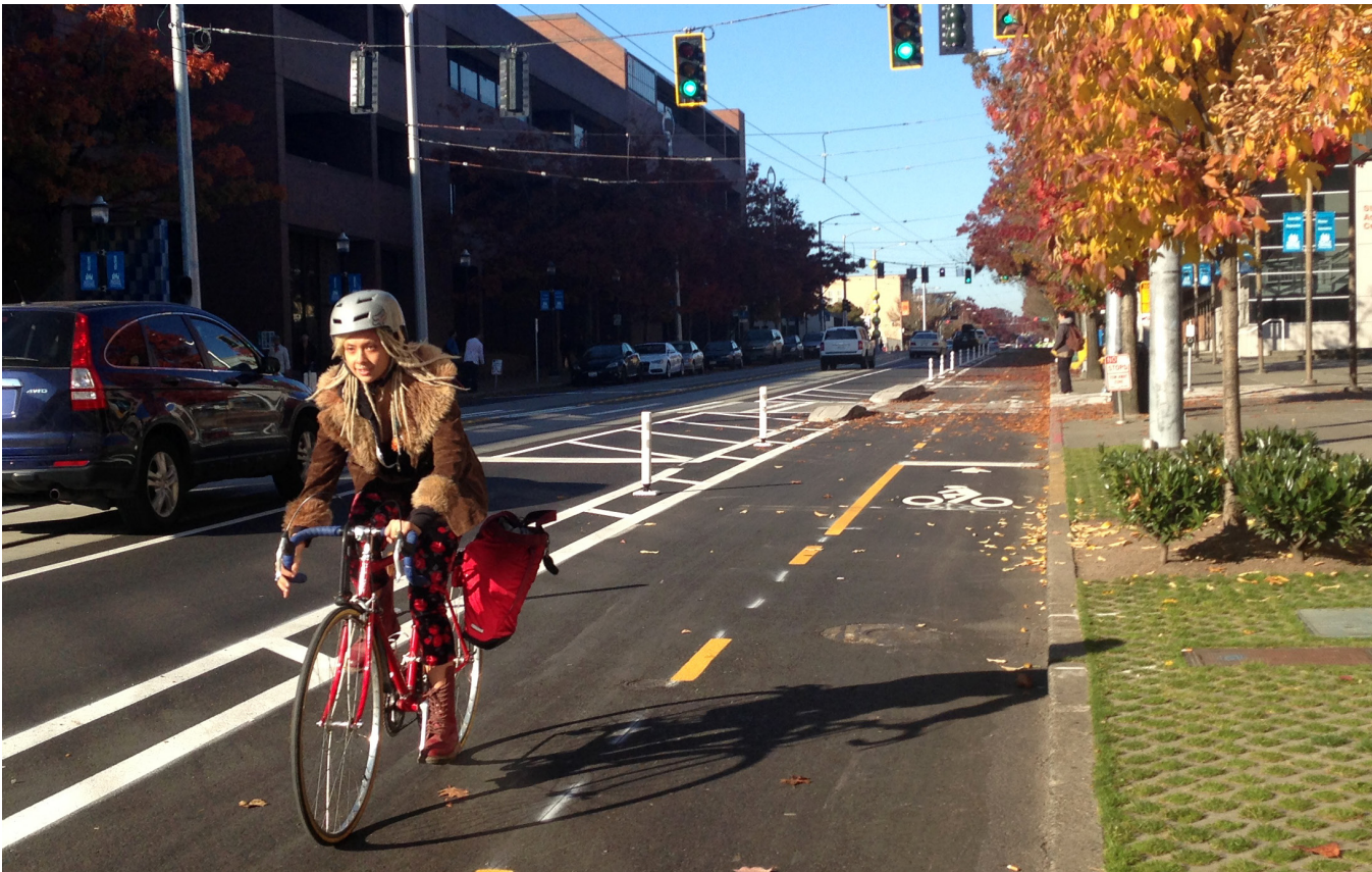
Seattle's newest bicycle infrastructure is a two way cycle track on Broadway. This is a way for bicyclists to travel with less conflict alongside cars or pedestrians.
