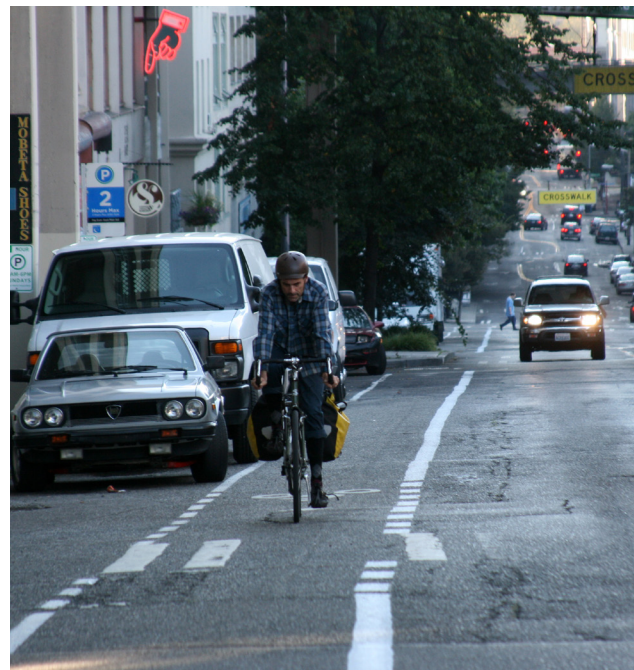
Climbing lanes provide a space for bicyclists on hills while allowing motor vehicles to pass.
