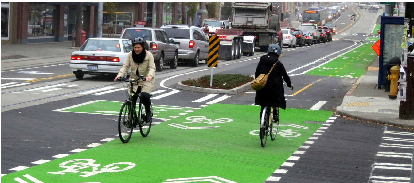
The cycle track on Broadway provides a physical separation between motorized and bicycle traffic.
